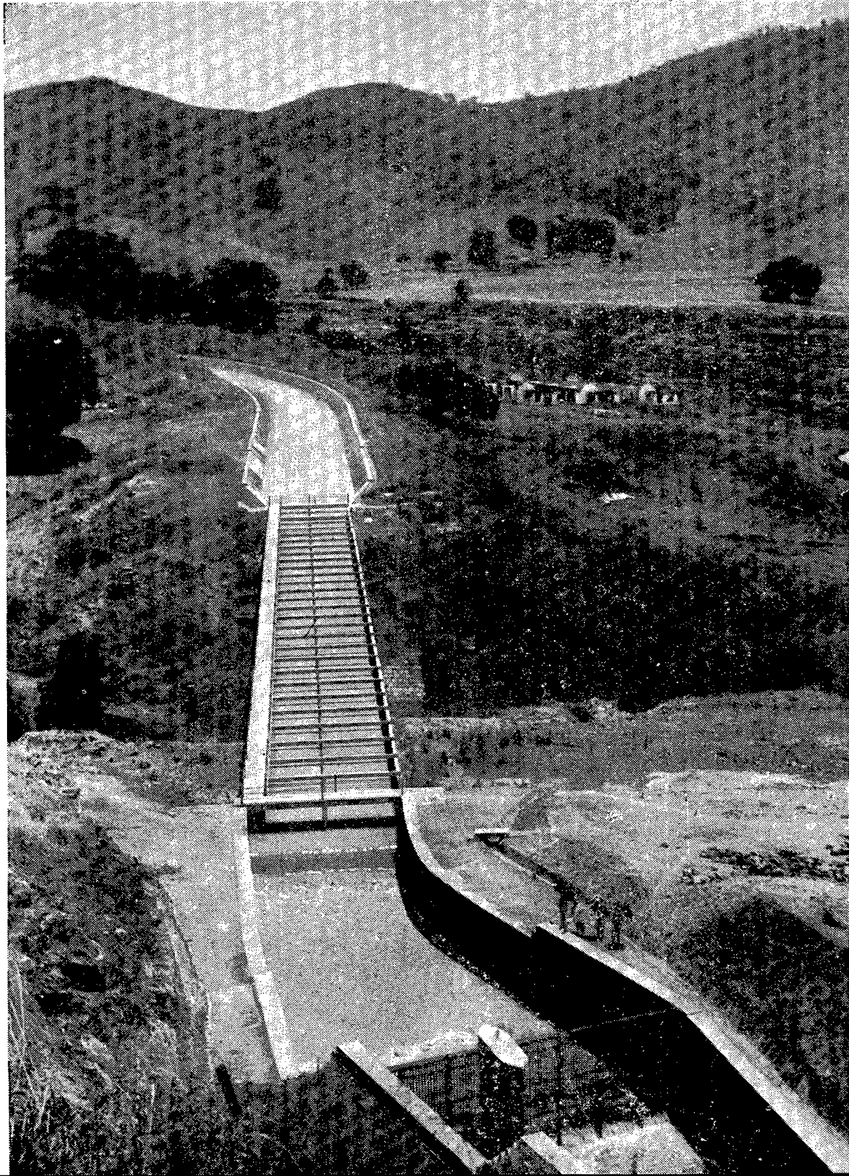
A concrete-lined irrigation channel of the Machkund Project, Andhra Pradesh
