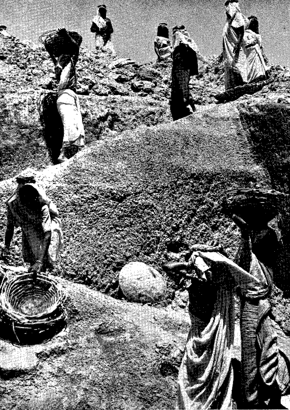
Work goes on to build a housing colony for Ranchi's labourers.
