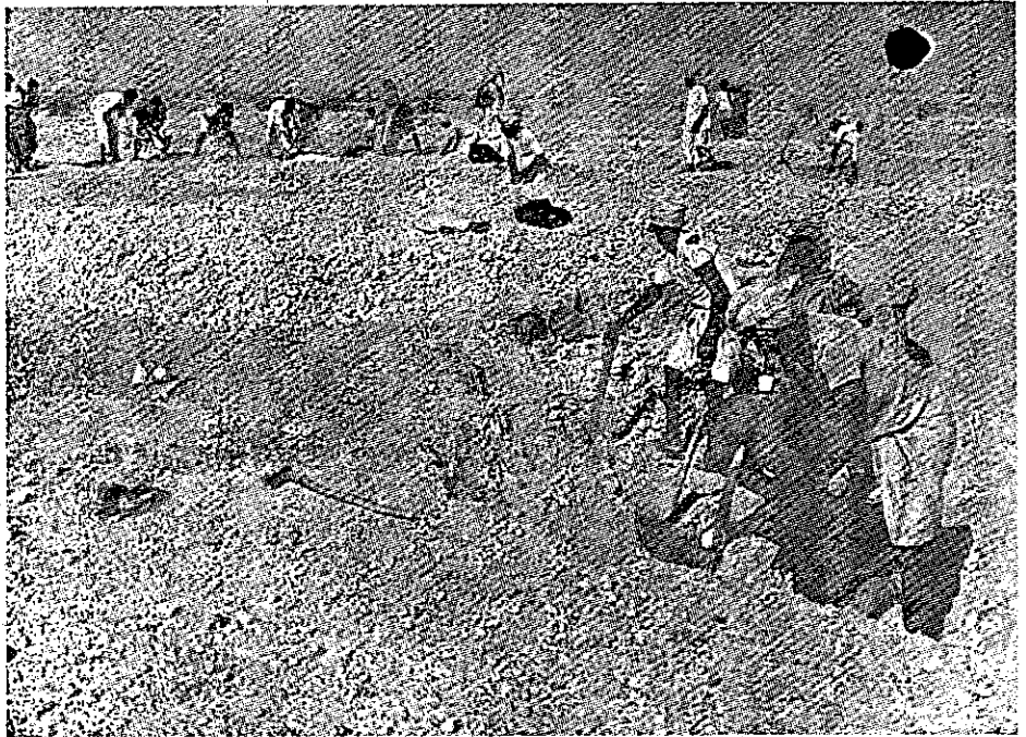
A road under construction
