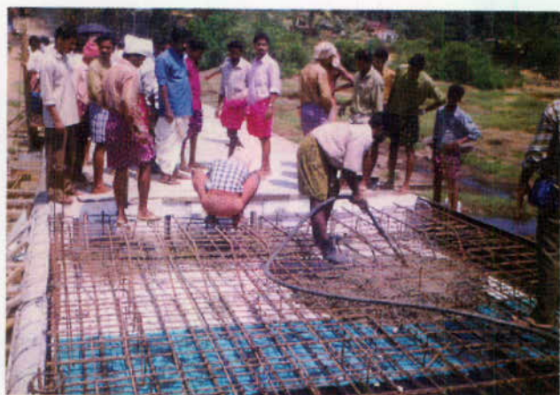
Improving Rural Infrastructure - Construction of Bridge
