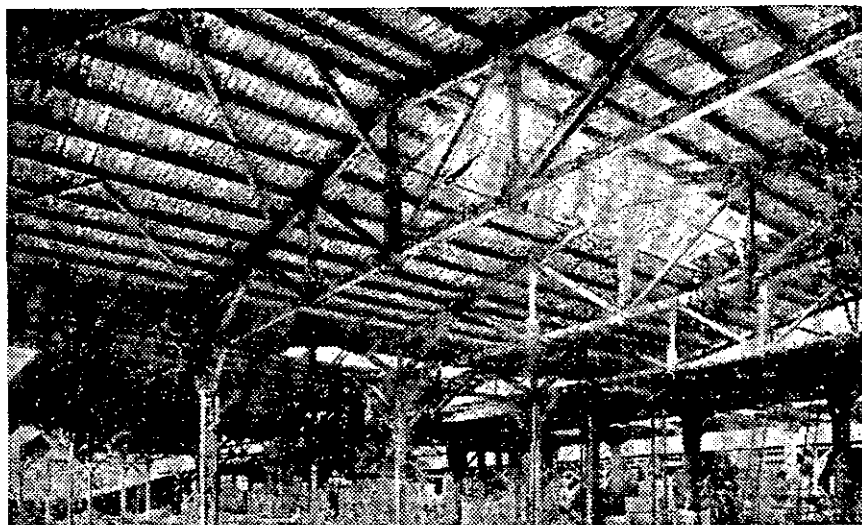
Laminated arched roof for a sports arena
