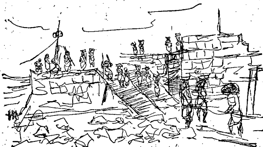
Nagarjunasagar—which lays emphasis on using more manpower than machinery
