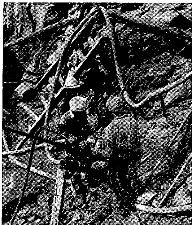
Pneumatic drill being used for cleaning rock face at Bhakra
