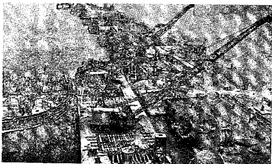
A partially built crib five metres high and 1,500 tonnes in weight is being launched at Visakhapatnam. It was later tugged to the site in mid-ocean, to be built to its full 23 meters height. The ore berth of the outer harbour is built upon eight such cribs.
