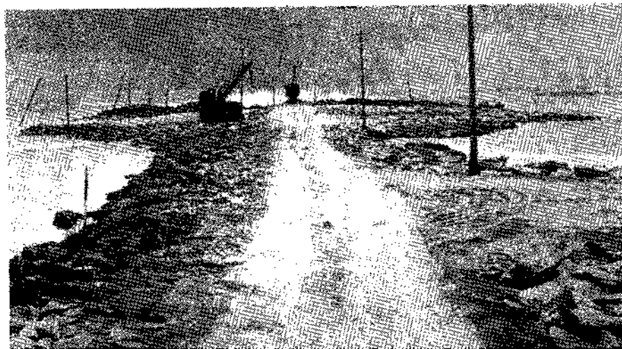
A View of the finished breakwaters
