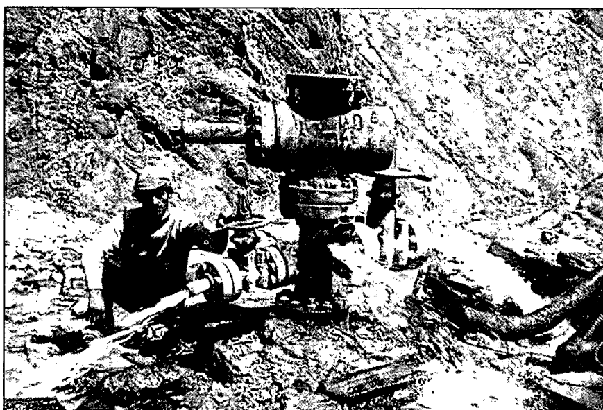
Hot Water (66½°C) discharge from 728 m deep borehole in Tapovan, Chamoli (Uttaranchal)
