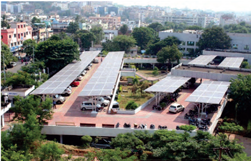
Solar Rooftop on Municipal Parking Lots at Visakhapatnam
