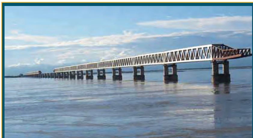
The Bogibeel Bridge, the longest Rail-cum-Road Bridge of the country running 4.94 km in length across river Brahmaputra near Dibrugarh in Assam has been commissioned, connecting Assam and Arunachal Pradesh. Dedicated to the nation by the Prime Minister on 25th December, 2018 the bridge has double line track with three-lane road and 74 km of total railway track.
