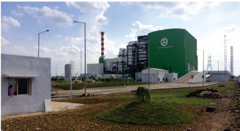
Jabalpur Waste-to-Energy Plant on PPP mode
