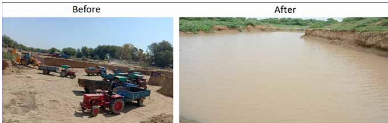
Figure 9: Before/ after images of water conservation work in Ranej village, Banaskantha. Increase in storage capacity by 5 lakh cubic feet.
