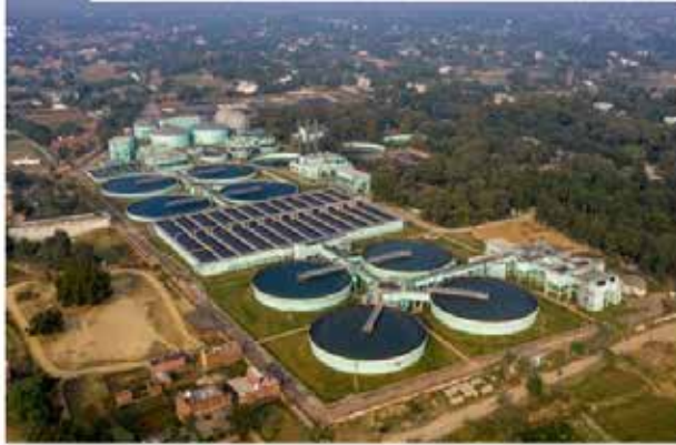
140 MLD State of the Art STP at Dinapur, Varanasi
