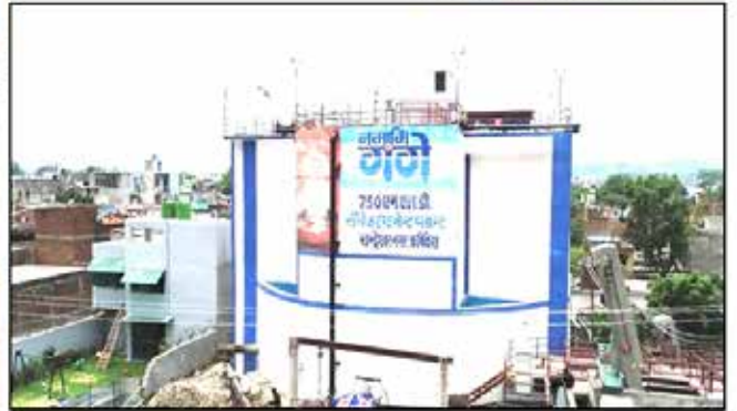
7.5 MLD STP, Chandreshwar Nagar, First four storey STP
