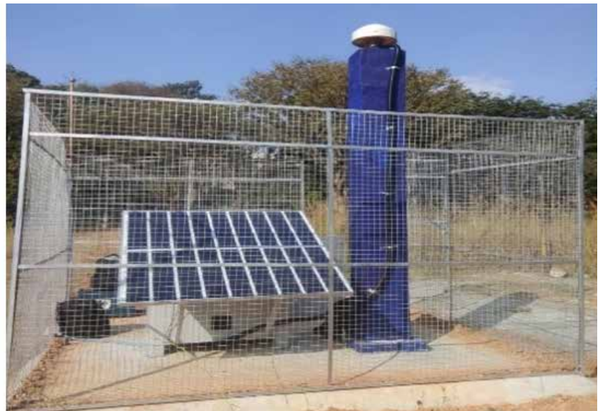
Drone-based survey and CORS station
