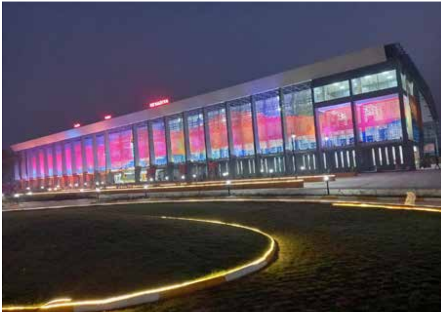
Kevadiya Railway Station in Gujarat is equipped with energy efficient lighting and is the first railway station with a Green Building Certification
