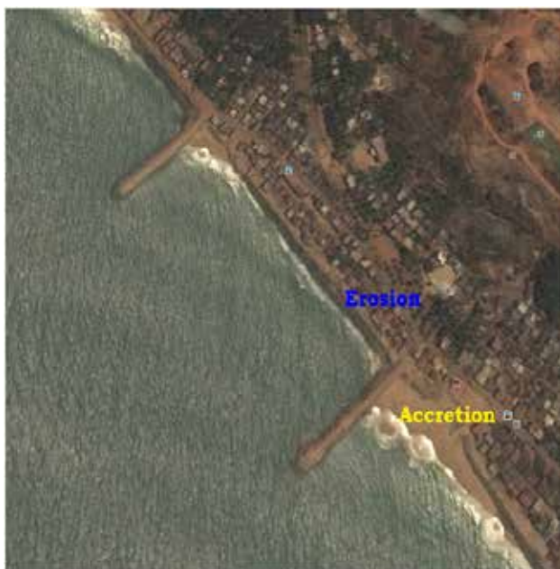
Groynes, a rigid hydraulic structure built perpendicularly from an ocean shore (in coastal engineering) or a river bank
